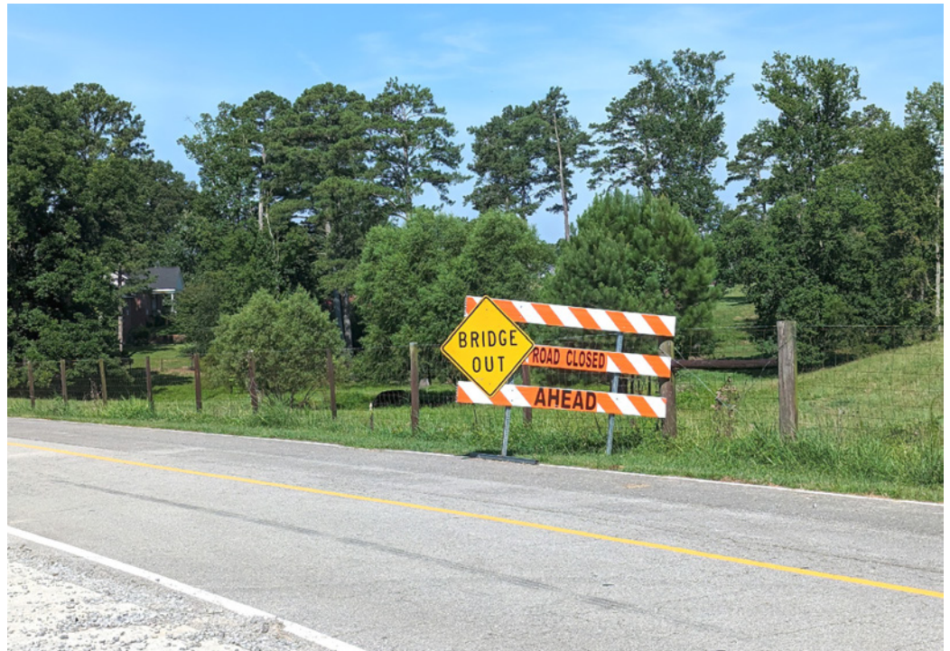
Ongoing construction for the new bridge on Lick Creek Road
